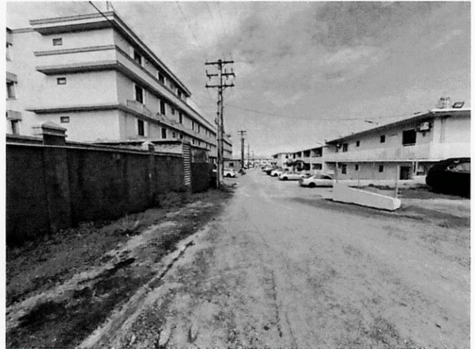
Westbound view of Sali Lane, the subject is to the right of the photograph (note the parking area within the 20' access easement portion).
